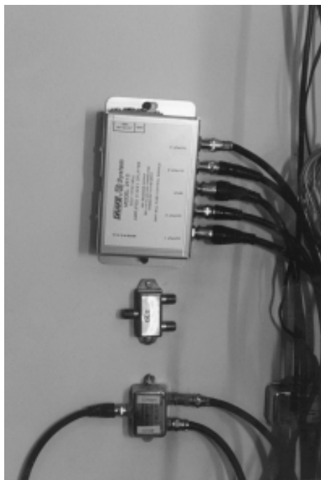
Drake Amplified four-way splitter which replaces the two-way splitter below it. (Photo courtesy the Guilty Party)
