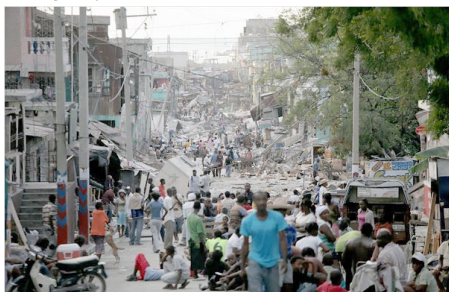
Destruction following the earthquake in Haiti. (Courtesy: SATERN)
