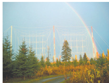
The Sterba curtain array is a chain of identical collinear elements as in the TCI Dipole Array at KNLS, Anchor Point, Alaska. The initial elements are shown here as a center-fed antenna, although it can be fed at other points as well. (Courtesy: World Christian Broadcasting)
