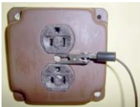
Wall outlet screw had to be loosened a bit to get clip to "bite."
