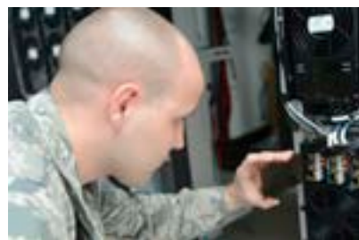
Senior Airman Jared Arledge opens a back compartment of the tower on the trunking system at MacDill Air Force Base Fla. The Trunked Radio System is a computer-controlled two-way radio system that allows sharing of radio frequency channels among a large group of users. (U.S. Air Force photo by Airman 1st Class Vernon Fowler)
