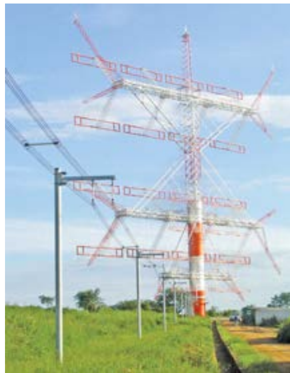
The Thomson HD-RCA Rotatable Antenna System delivers high power in a tight beam at HF. (Courtesy: Thomson)
