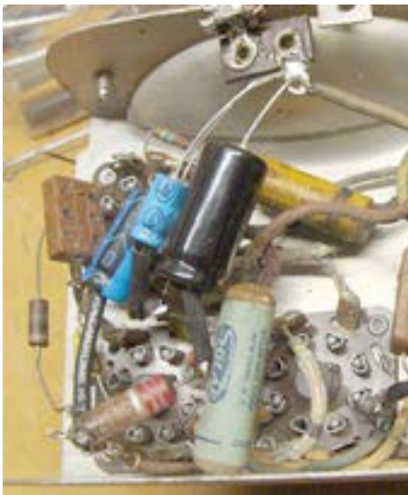
Once proper operation of the radio was verified, the electrolytics were installed permanently.
