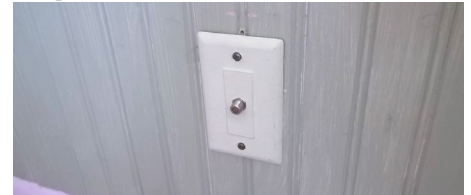
Photo 4. Wall plate with F connector for attachment to FTA radio. Tidy installation keeps me in the XYL's good graces.
