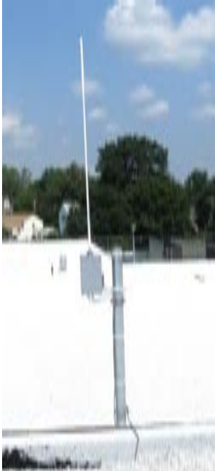
The free radiating Part 15 AM transmitter atop the McMahon main campus building. The transmitter was fitted with a short whip antenna during initial field strength testing.
