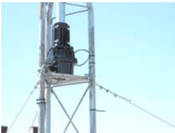
Expertly installed at W7MRE (The American Museum of Radio and Electricity in Bellingham, WA), this Yaesu G800-SA rotator (a best buy in this year's MT Buyer's Guide), rated for a beefy 17 square feet of wind load) loafs along while aiming the club station's Traffie Technology Hex-Beam antenna, which has a wind-load rating of less than 5 square feet. Note the rotator shelf (see text). (Photo by, and courtesy of, Phil Terzian, AE6K.)
