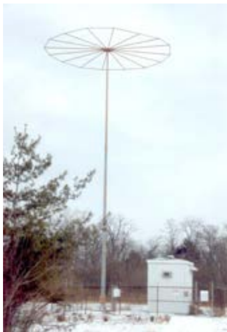
Typical NDB, MDE/379 kHz in Cincinnati, Ohio, this site uses one of the newer "tophat" style antennas. (File Photo)
