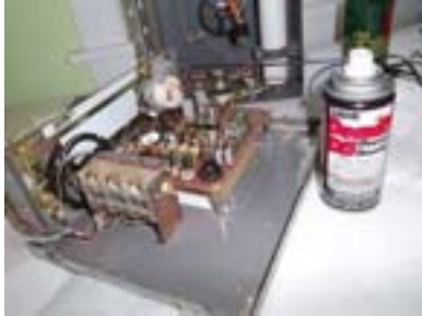
Coastal Navigator chassis cleaned and ready for checkout.
