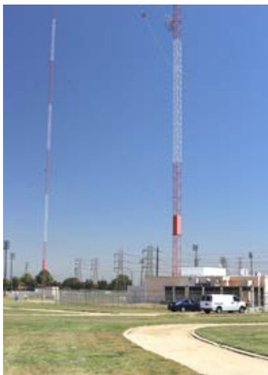
Figure 1. An overall view of the KNX transmitter site today, showing the transmitter building, main tower (right, rising out of the building), auxiliary tower (left), and security fencing around all installations. The site's layout in 1965 was substantially the same as today. A public park now surrounds the facility; both it and the auxiliary tower did not exist in 1965.
