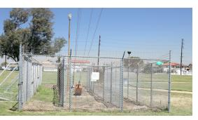
Figure 2. The main tower's north guy earth anchor today. One of the guy wires at this anchor was severed by saboteurs in 1965. Note the double level of fencing now surrounding the anchor point. No access barriers or alarms existed in 1965.
