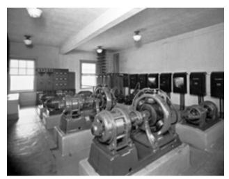
The generator room of the General Electric station contained nine motor-generator sets. These supplied current for heating the filaments of the tubes, plate potential for the power amplifiers and the 600 meter commercial transmitter, bias potential for the amplifier and modulator tubes, and excitation for the various generators. These machines were all in duplicate, thus assuring a continuous program in the event of failure.
