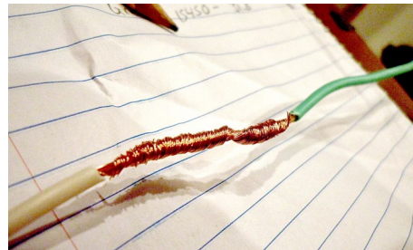
Use a strong Western Union Splice to join pieces of antenna wire.
