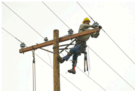
This photo of a Utah lineman repairing a damaged power line in the aftermath of Hurricane Rita always catches my attention. I'm not an expert on government regulations regarding lineman safety practices (so this may be completely compliant), but the use of the single "around the waist D-ring belt" is not suitable for antenna tower work. In this configuration, during a slip or fall it's easy to flip upside down or suffer a broken back. (FEMA photo by Marvin Nauman courtesy of Wikimedia Commons).
