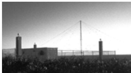
DGPS stations like this one in Cape Ray, Newfoundland, broadcast high precision correction signals to GPS users in the vicinity (file photo).
