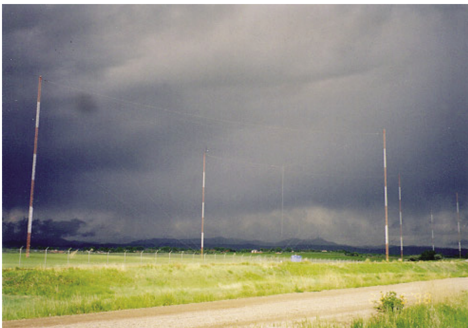
WWVB's 60 kHz antenna system cranks out 50 kW (ERP) from its 38 kW transmitter in Boulder, CO. (Courtesy NIST)
