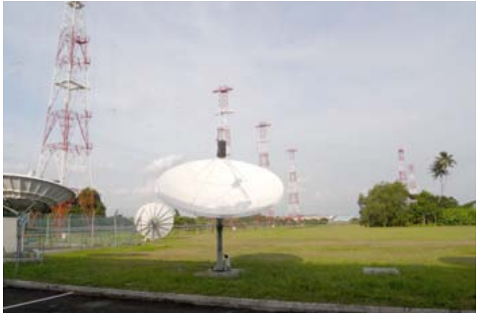
Satellite dishes to downlink BBC programming are in the foreground with the shortwave curtain antenna in the background. Note the elevation of the dishes are nearly straight up this close to the equator.
