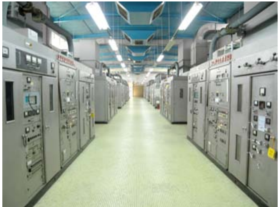
The transmitter hall with rows of 100 kW and 250 kW Marconi transmitters. These are the originals that were sent to Singapore in 1964 and installed in 1965. Tam told me this station could operate for another 40 years with no problems. What you don't see are three 50 kW Marconi transmitters in the back that are used for backups in case anything was to happen to these giants
