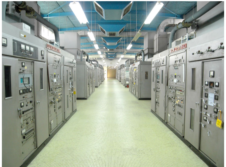
The transmitter hall with rows of 100 kW and 250 kW Marconi transmitters. These are the originals that were sent to Singapore in 1964 and installed in 1965. Tam told me this station could operate for another 40 years with no problems. What you don't see are three 50 kW Marconi transmitters in the back that are used for backups in case anything was to happen to these giants
