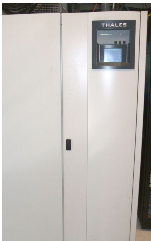
A Thales UHF digital TV transmitter. (I'll bet you thought it would be bigger!)
