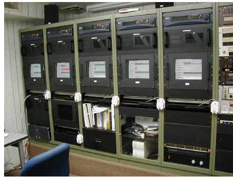
Controls for new 250,000 watt, DRM-capable, Thomson transmitters at TRW's Guam site. (Courtesy: TRW)
