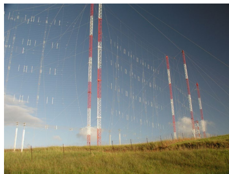
Massive curtain antenna just one of four beamed at Australia, Southeast Asia, India, and China. (Courtesy: TRW)
