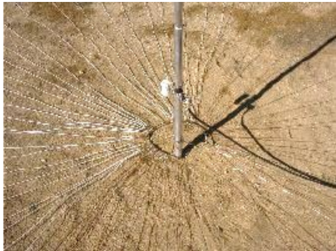
A more robust radial arrangement at the base of a vertical.
